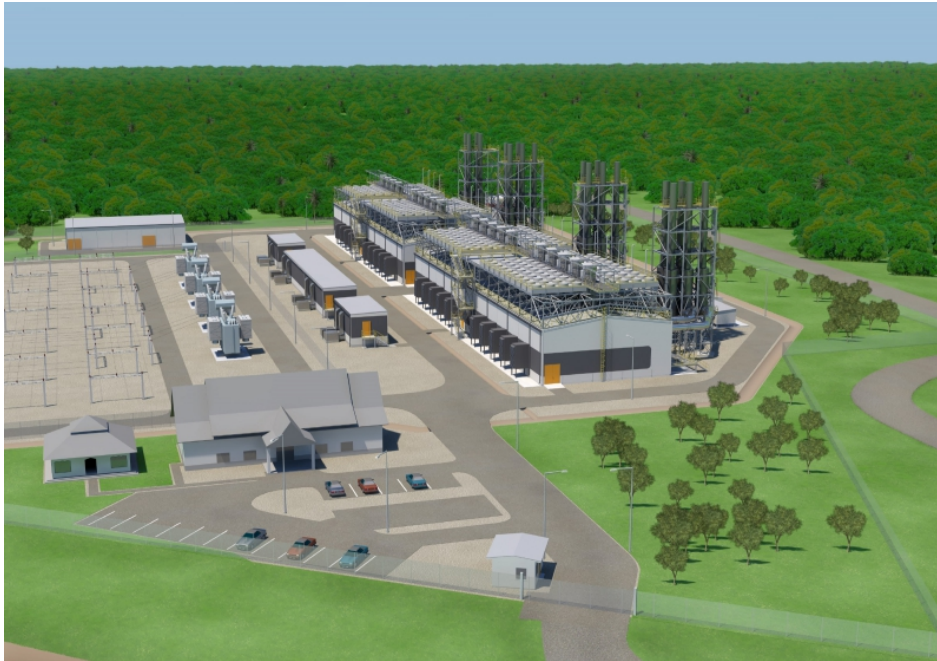
Illustration of the 184 MW Arun gas power plant that Wärtsilä will deliver to Indonesia.
